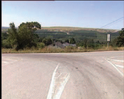
Old markings confuse pedestrian and motorists. Redundant reflective markers misguide motorists.
