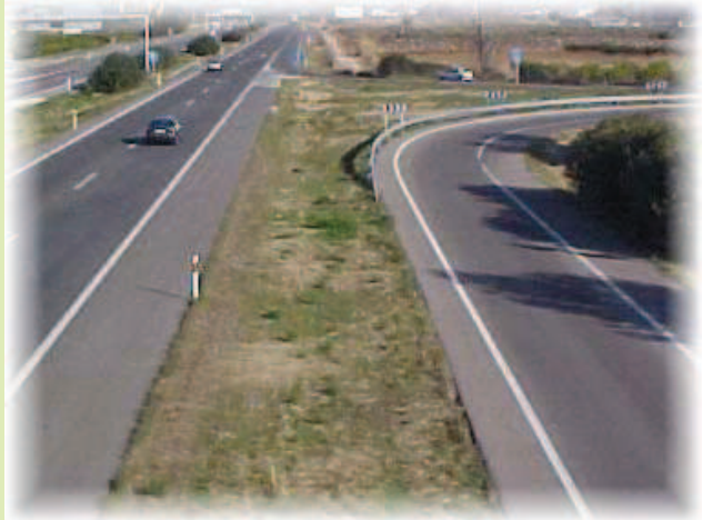
Short distance between central lines and service road.
