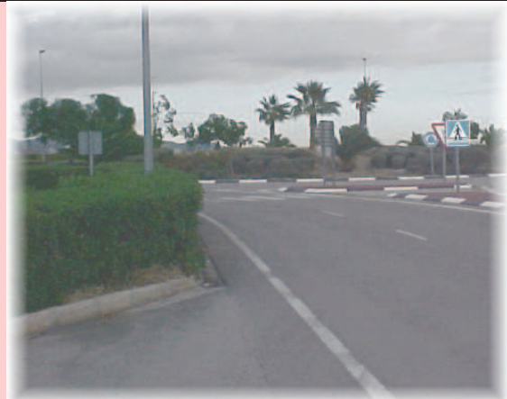
Service road too close to the roundabout
