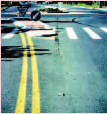
Old markings confuse pedestrian and motorists. Redundant reflective markers misguide motorists.
